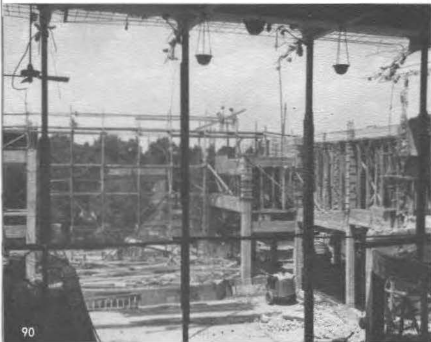
Early Stage of Auditorium Construction.
