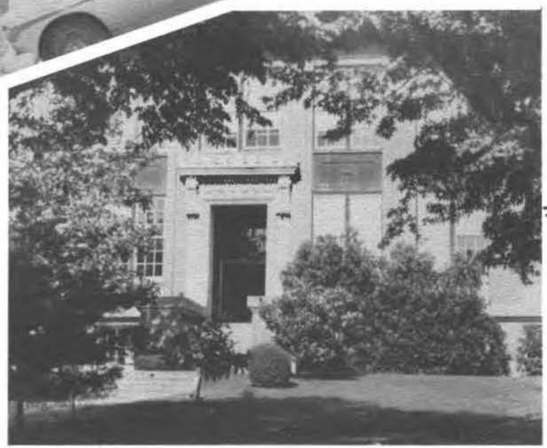
ADMINISTRATION BUILDING SIDE VIEW
